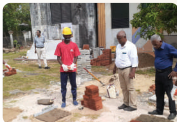
Two batches of NVQ Level 3 and 4 qualifications completed for masons and tilers in partnership with CIDA
