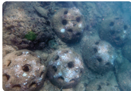
Reef balls at the Walduuwa site showed strong survival and no structural damage
