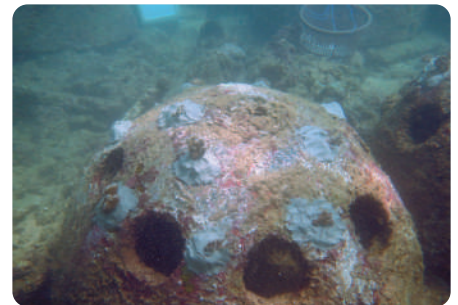
Reef balls at the Walduuwa site showed strong survival and no structural damage
