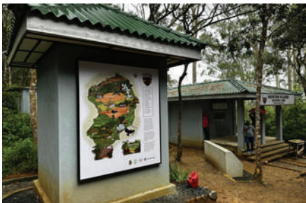
The new administrative complex is complete with all visitor amenities
