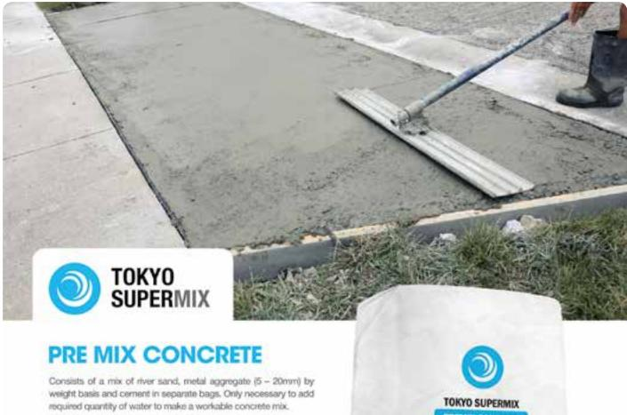
Equivalent concrete grade is G20. TOKYO SUPERMIX PREMIX CONCRETE can be used for slabs, driveways, pavements etc. Available in 50kg bag. 30 bags can cover an area of 10ft x 10ft x 0.25ft.
