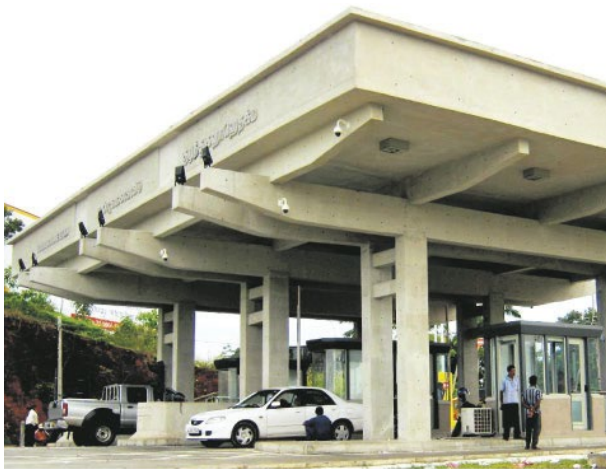
Toll Gates of Southern Expressway Kurundugaha-Hathakma
